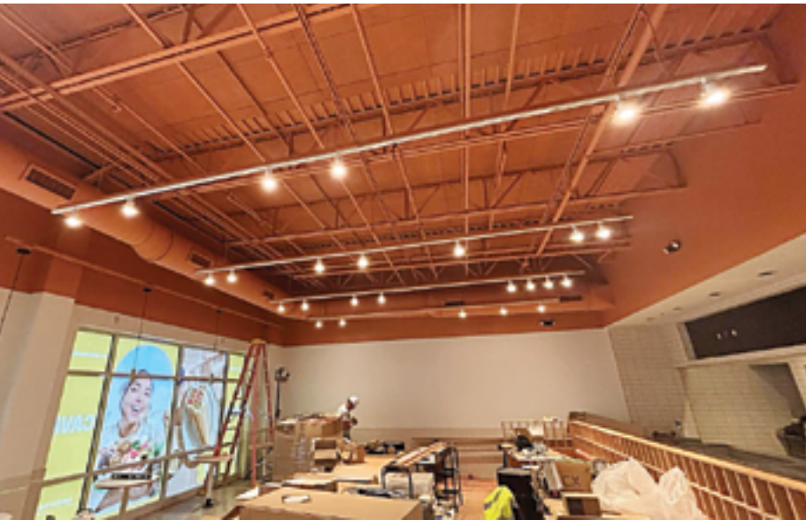
Inline Painting works on an interior painting project.
